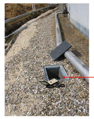
The sensing cable is visible as it exits the blue slotted pvc conduit.
