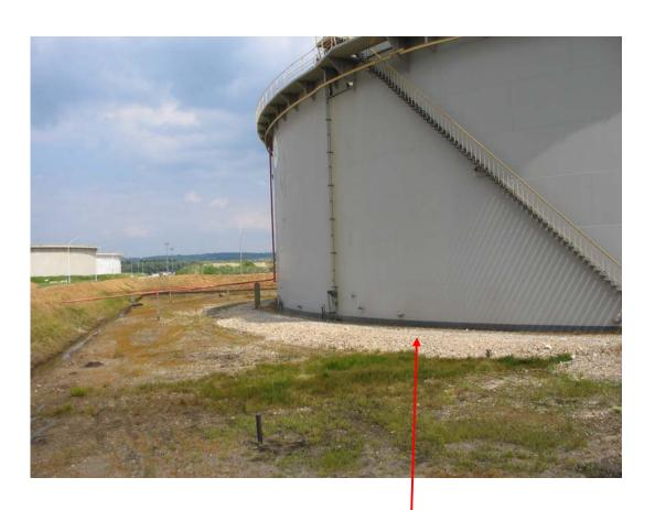
The 4 crude oil tanks are surrounded by 1 km of T5000 cables buried 50 cm deep in the ground.
