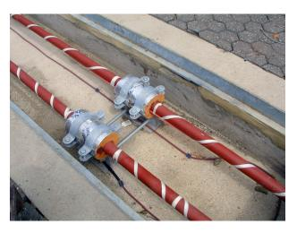
TraceTek TT5000 cable clipped to the base of the concrete trench close to the pipe, prior to the insulation been fitted.
