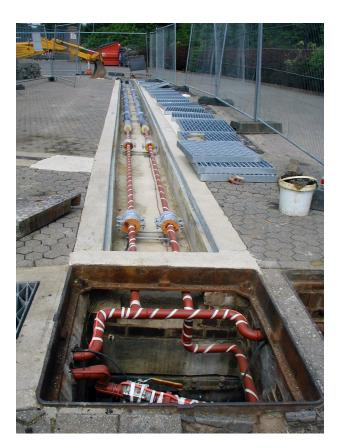
TraceTek Leak Detection and Locating Systems can monitor miles of single wall buried pipelines for fuel leaks, provide a precise location of a small developing leak, close valves before it becomes catastrophic, and interface with a pipeline monitoring system or BMS.
