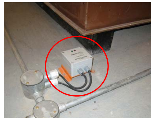
AT-OPSEN Optical Sensor placed on all four corners of the tank to provide optimum coverage.
