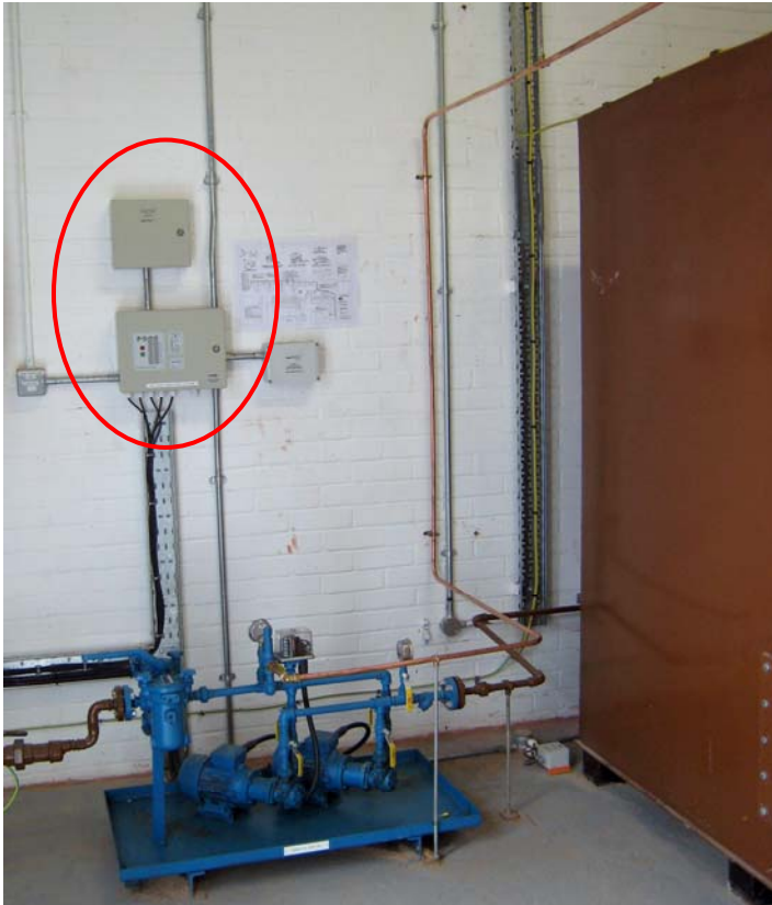
AquiTron Multi Zone Alarm Panel with Battery Back-Up, monitoring 5 zones/rooms which have been fitted with a combination of Optical Sensors and TT5000 Sensing cable.
