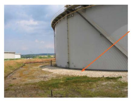
Product: TraceTek TT5000 sensing cableApplication: Sensing cable directly buried in a trench looping around the perimeter of the tank.Site: France
