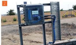
1) 4 x TTC-1 controller with MTL 7767+ Zener barriers. 2) wired to junction boxes with branch connectors local to the tanks proving a centralised monitoring system.
