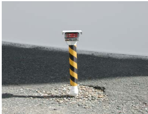
The TT-FLASHER Leak Alarm Module monitors for leaks at a storage tank facility in Brisbane, CA.
