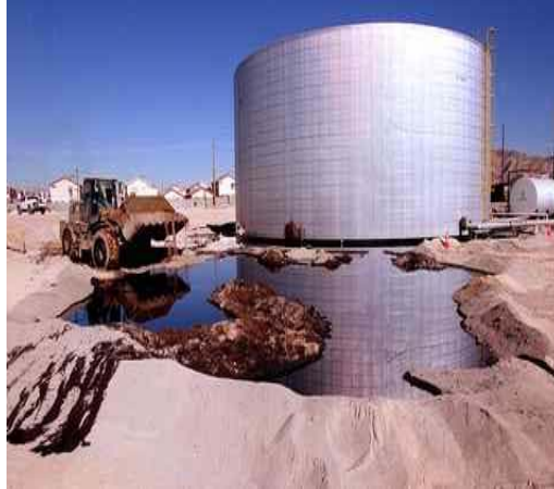
Petroleum product leakage from an above ground storage tank threatens the health and safety of a near by residential neighborhood with environmental damage and contamination.
