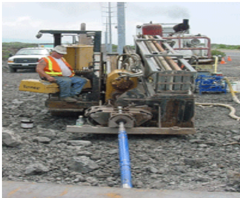
Directional drilling bores below the tank bottom for installation of the Schedule 80 PVC slotted conduit.
