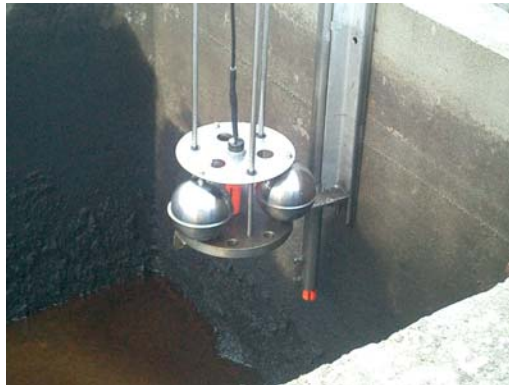
Mixed floating and fixed TT-FFS installation in a sump
