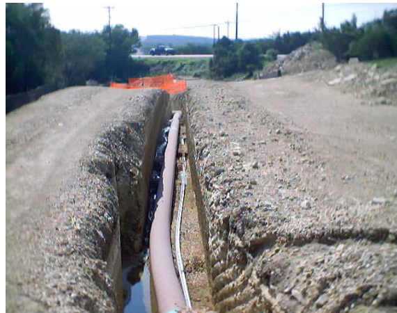
TraceTek TT5000 Sensing Cable installed inside slotted PVC conduit along side a single wall buried pipeline
