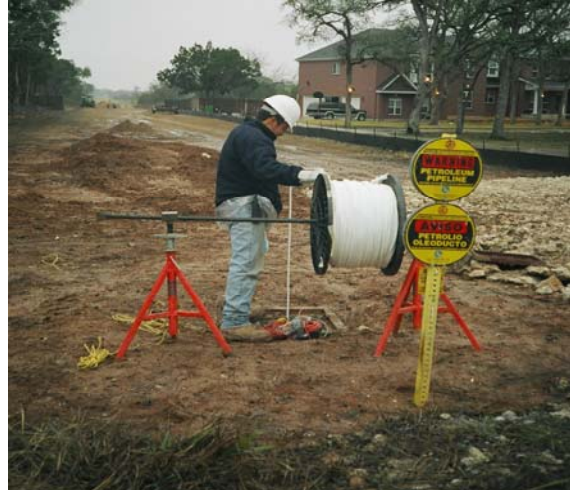
TraceTek Leak Detection System being installed in a 12 km "High Consequence Area" along the Longhorn Pipeline in Austin, TX
