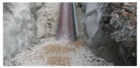
Shown above is a typical installation showing the main fuel oil carrier pipe and the laser slotted PVC conduit located side by side in the trench. Standard backfill and compaction is used to cover the pipe and conduit. TraceTek Direct Burial fuel oil sensor cables are later pulled into the conduit.
