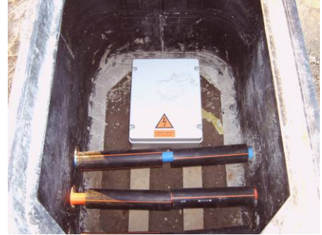
Typical design of sensor cable and access shaft with connecting box
