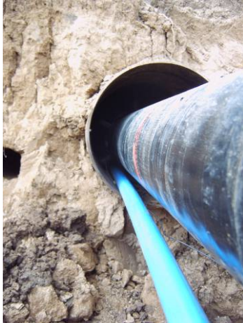
Blue conduit with sensor cable installed in a coated pipe under a street.
