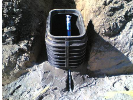
Typical design of sensor cable and access shaft with connecting box
