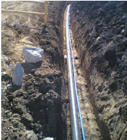
TraceTek Sensor cables are installed parallel to the pipeline by pulling through the permeable blue conduit shown.
