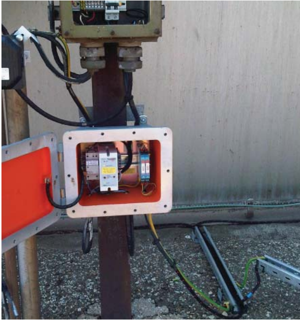
TraceTek TTC-1 SIL2 controller housed local to the sensor within an Exd enclosure with two zener barriers.
