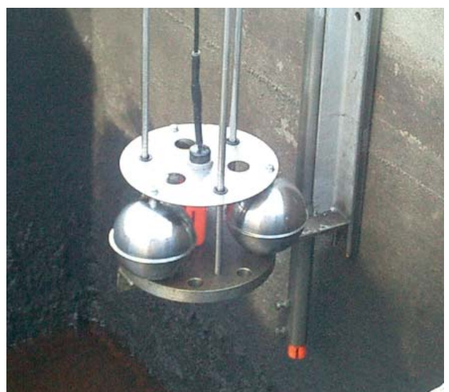
TraceTek Fast Fuel Sensor (TT-FFS) installed within sump to detect varying water levels.
