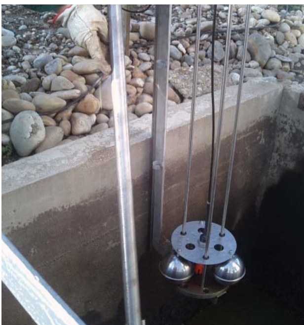
TraceTek Fast Fuel Sensor (TT-FFS) installed within a rain water outfall.
