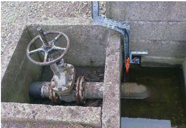
TraceTek Fast Fuel Sensor (TT-FFS) installed within a rain water outfall.
