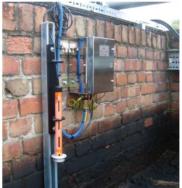
TraceTek Fast Fuel Sensor (TT-FFS) attached to an adjustable height wall bracket to detect a catastrophic leak within a bund.
