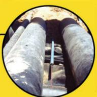
If your business involves the transportation, storage, processing or consumption of hazardous fluids, the possibility of a leak must be considered. **TraceTek**® provides a leak detection system tailored to your needs.
